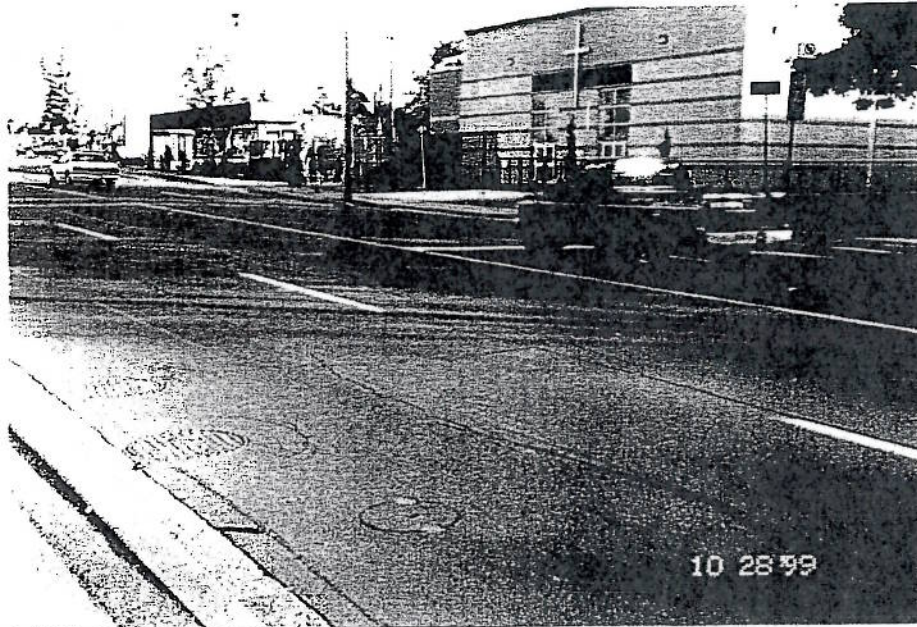
Photo 6 – Kennedy Road reinstatement in October 1999.
